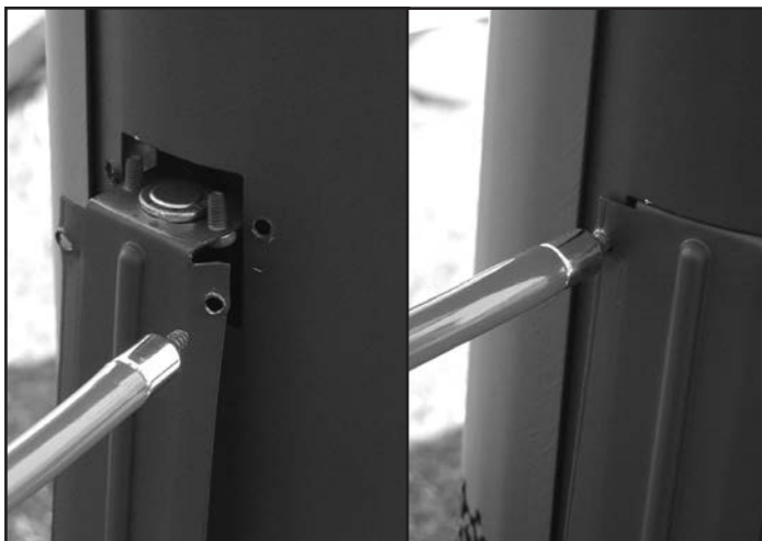
Figure 55: Spill switch installation.
