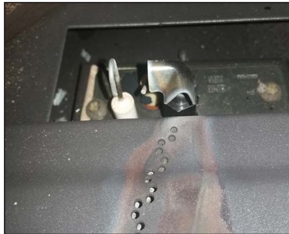
Figure 21. Correct Pilot
